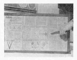
To permit trouble-free expansion in the future, pictorial wiring diagrams and instructions for tweeter and tweeter control connections are printed on cabinet's back.
